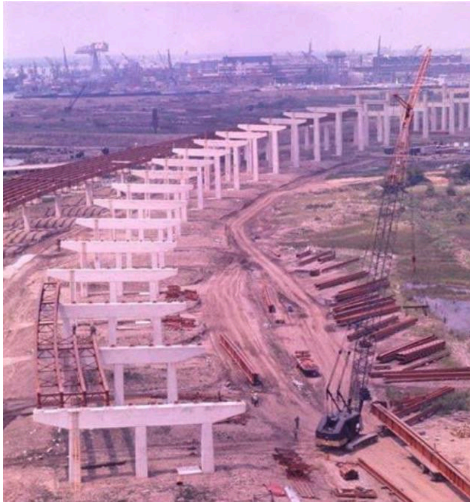
Construction of I-95, near Philadelphia, circa 1970.
