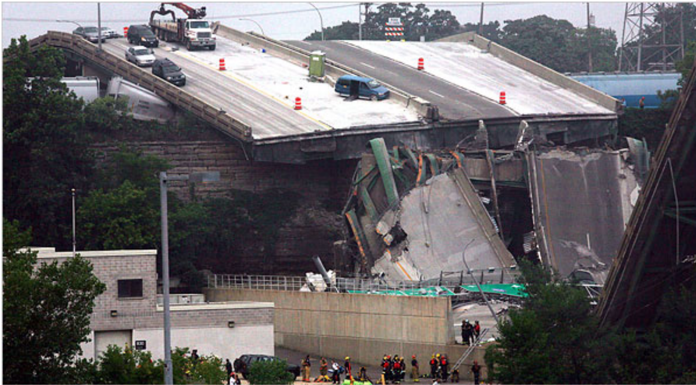
Collapsed I35 W. Mississippi Bridge, August 1, 2007.
