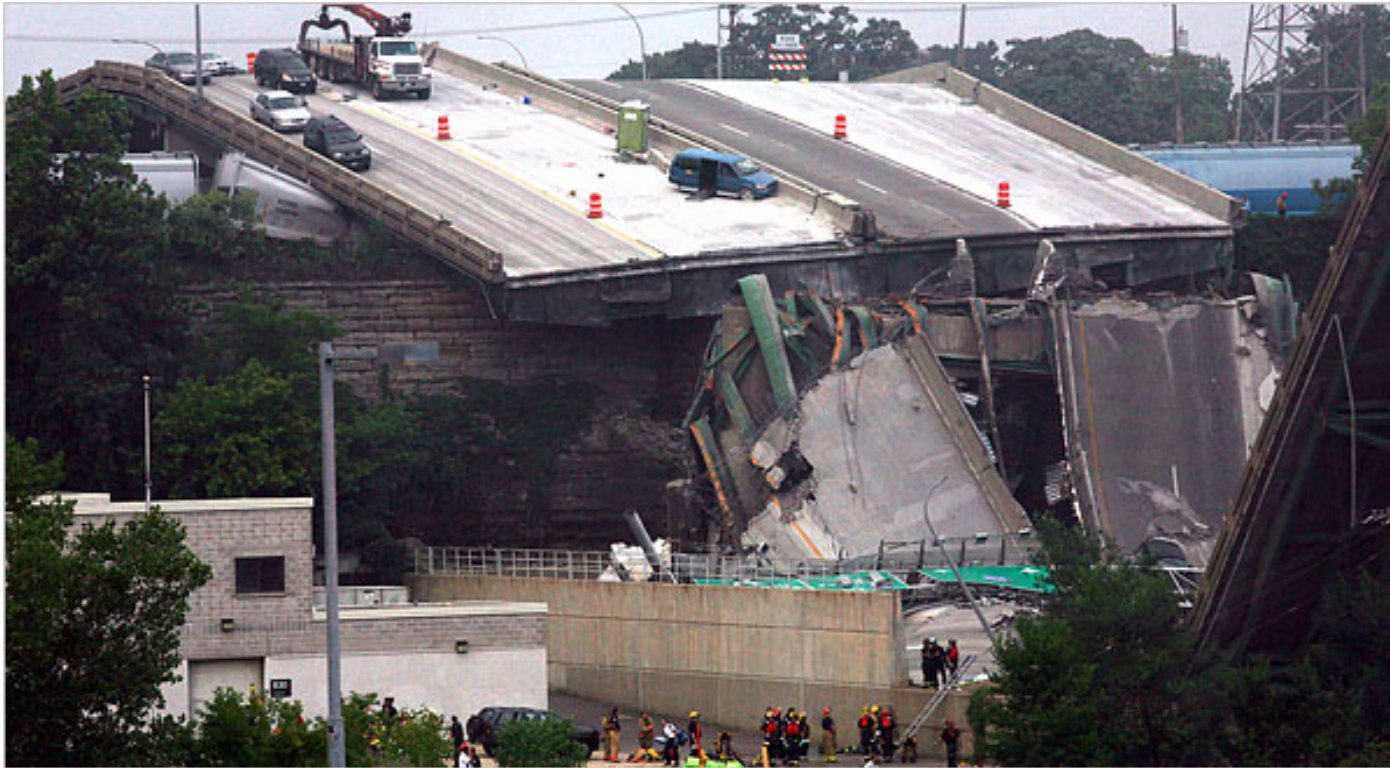
Collapsed I35 W. Mississippi Bridge, August 1, 2007.
