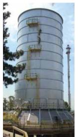
▲ Figure 4. Enclosed ground flares shield the surrounding community from radiation and noise. Here, an enclosed ground flare is seen with an elevated flare in the background.
